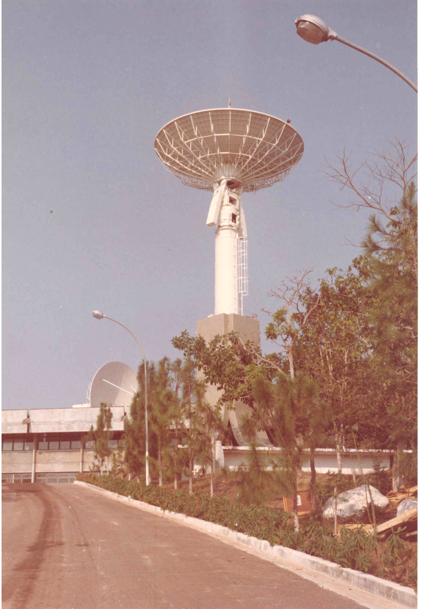
Fig. 1 - New antenna (S and X bands) at Cuiabá Station.
