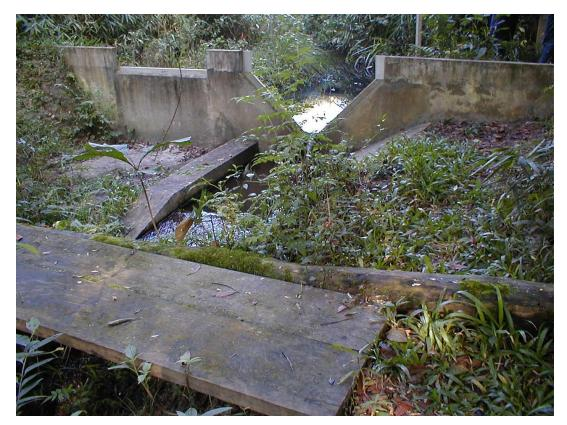
Figure 3a. Weir installed at the PEFI stream basin (Forti, 2000).
